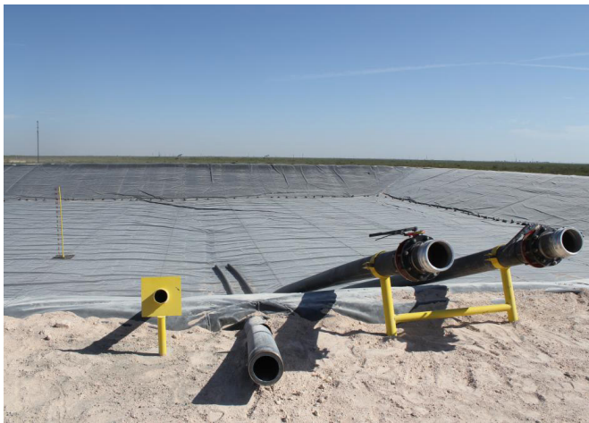
Figure 2. Fully outfitted storage pit.
