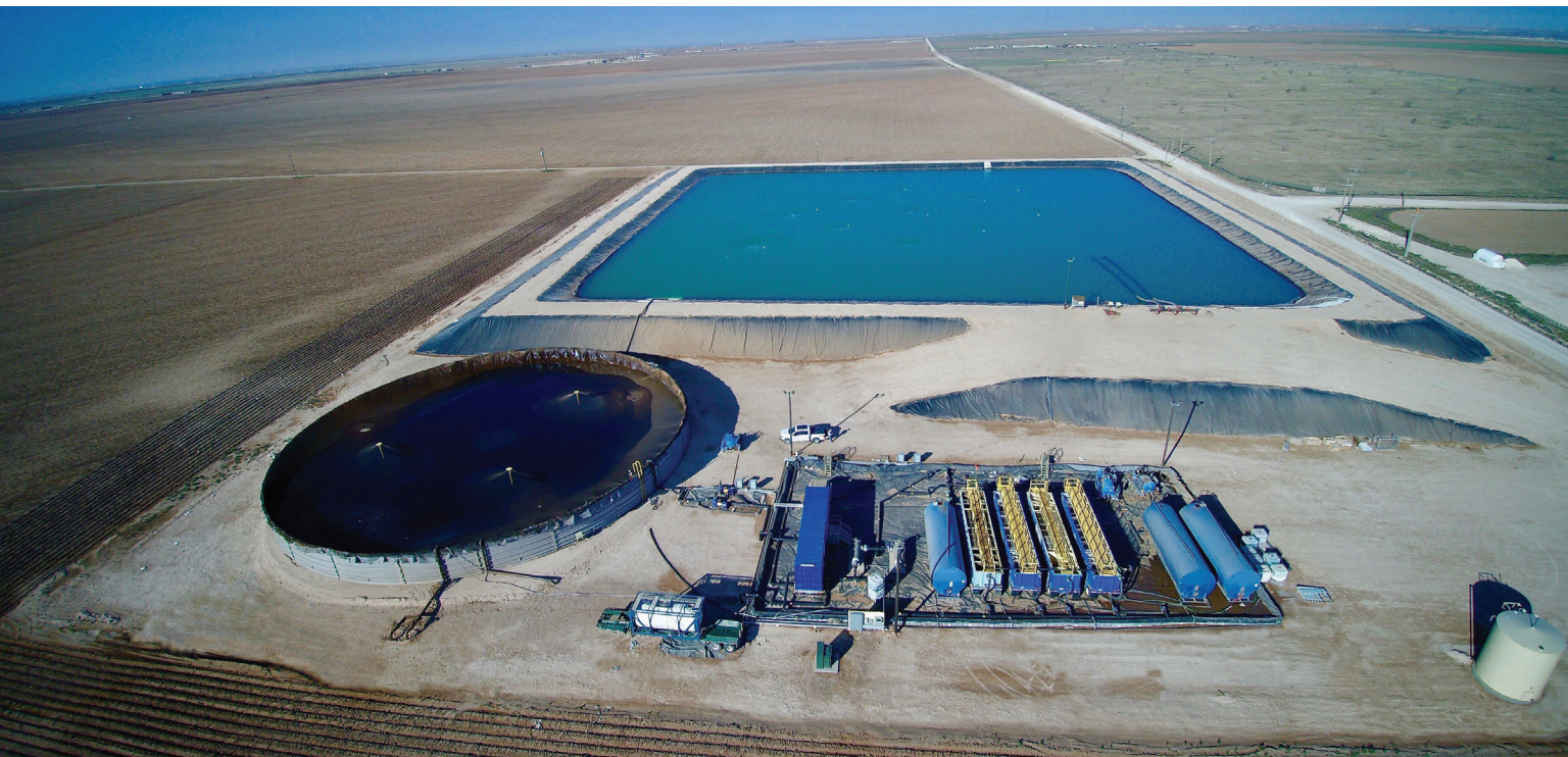
The SWAT system uses real-time monitoring and PLC control technology to provide operators with 24/7 access to their water recycling operations. This allows a transparent, on-demand view of the chemistry, treatment volumes and water quality being delivered from the system. (Source: TETRA Technologies)
